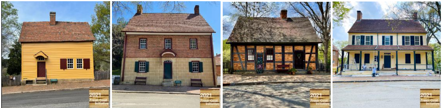
(left to right) Completed Fresh Coat Projects: Miksch House c. 1771, Winkler Bakery c. 1800, Fourth House c. 1767-68, and c. 1816 Tavern street porch
