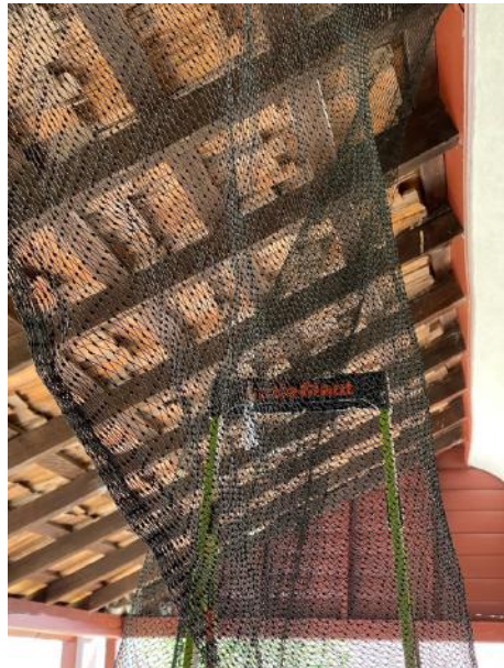
(left to right) The Back Porch of Winkler Baker, a quiet resting place for our visitors, has been long neglected because birds and critters would nest up in the wood-shake roof structure, resulting in many animal waste and bird droppings covering the surfaces below. As part of our Fresh Coat Initiative, we have installed barely visible preservation netting to keep out these animals. Now the back porch can become a clean, welcoming spot for our guests.
