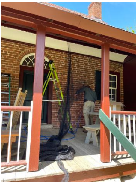
(left to right) The Back Porch of Winkler Baker, a quiet resting place for our visitors, has been long neglected because birds and critters would nest up in the wood-shake roof structure, resulting in many animal waste and bird droppings covering the surfaces below. As part of our Fresh Coat Initiative, we have installed barely visible preservation netting to keep out these animals. Now the back porch can become a clean, welcoming spot for our guests.
