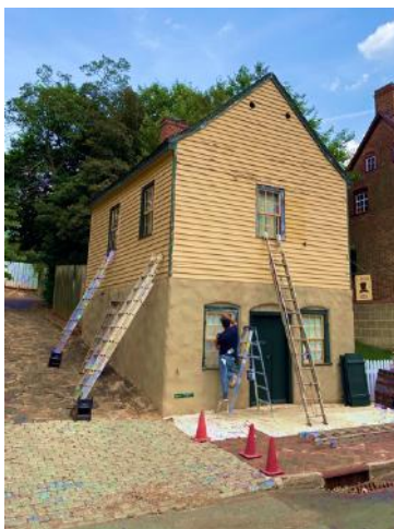
(left to right) The Butner workshop & store building is the latest historic structure to be worked on. Although a small building, the wood repair needed to the exterior clapboard (although cedar) was more extensive than anticipated. Due to selective wood clapboard repair, we paid particular attention to the appearance & location of the visible handmade nails. Special thank you to Erik Skarzynski, Director of Facilities for project managing.
