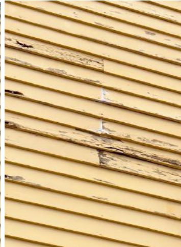
(left to right) The Butner workshop & store building is the latest historic structure to be worked on. Although a small building, the wood repair needed to the exterior clapboard (although cedar) was more extensive than anticipated. Due to selective wood clapboard repair, we paid particular attention to the appearance & location of the visible handmade nails. Special thank you to Erik Skarzynski, Director of Facilities for project managing.
