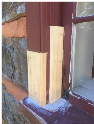
(left to right) Our Fresh Coat Initiative work includes the wood window repair and painting of the St. Phillips Log Church. As a fully reconstructed building, the material selection and replacement involve less restrictive parameters. Just as in the Butner Shop building, the selective wood replacement at the log church requires attention in the appearance of the location and type of nails. We are considering the repair of the “chinking” to become a public-facing preservation workshop. Thank you to Tony Bragg, Facilities Team, for his work on the window repair and painting.
