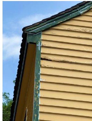
(left to right) The Butner workshop & store building is the latest historic structure to be worked on. Although a small building, the wood repair needed to the exterior clapboard (although cedar) was more extensive than anticipated. Due to selective wood clapboard repair, we paid particular attention to the appearance & location of the visible handmade nails. Special thank you to Erik Skarzynski, Director of Facilities for project managing.
