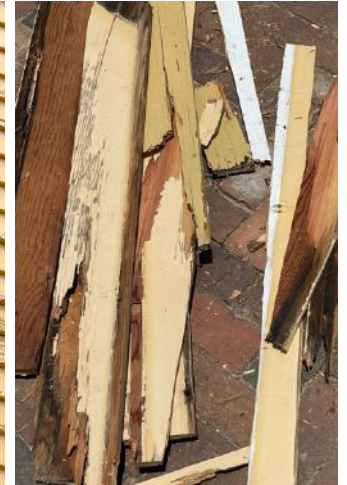
(left to right) The Butner workshop & store building is the latest historic structure to be worked on. Although a small building, the wood repair needed to the exterior clapboard (although cedar) was more extensive than anticipated. Due to selective wood clapboard repair, we paid particular attention to the appearance & location of the visible handmade nails. Special thank you to Erik Skarzynski, Director of Facilities for project managing.
