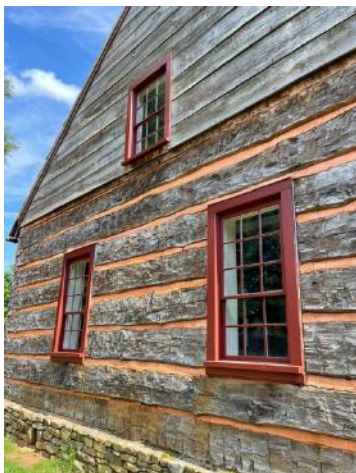
(left to right) Our Fresh Coat Initiative work includes the wood window repair and painting of the St. Phillips Log Church. As a fully reconstructed building, the material selection and replacement involve less restrictive parameters. Just as in the Butner Shop building, the selective wood replacement at the log church requires attention in the appearance of the location and type of nails. We are considering the repair of the “chinking” to become a public-facing preservation workshop. Thank you to Tony Bragg, Facilities Team, for his work on the window repair and painting.
