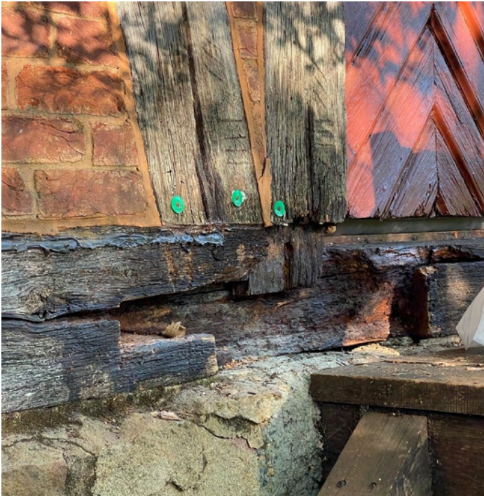
(Left to right) The orthwestern corner of the Fourth House was in need of considerable repair. Due to poor water drainage at the rear stair, an entire wood joint had rotted away from the sill timber. . . A dutchman repair was utilized to seamlessly patch the compromised joint. The handrail had also dislodged from the building and was failing. Each step of the restoration can be seen in these photographs. The final restoration is pictured below. This repair was primarily completed by joiner Ben Masterson with assistance from craftsman Blake Stevenson and the logistical assistance of Erik Skarzynski , Director of Facilities and Tony Bragg , Facilities Associate.
