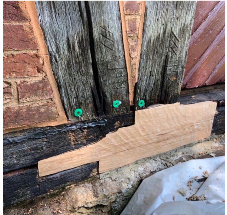
(Left to right) The orthwestern corner of the Fourth House was in need of considerable repair. Due to poor water drainage at the rear stair, an entire wood joint had rotted away from the sill timber. . . A dutchman repair was utilized to seamlessly patch the compromised joint. The handrail had also dislodged from the building and was failing. Each step of the restoration can be seen in these photographs. The final restoration is pictured below. This repair was primarily completed by joiner Ben Masterson with assistance from craftsman Blake Stevenson and the logistical assistance of Erik Skarzynski , Director of Facilities and Tony Bragg , Facilities Associate.
