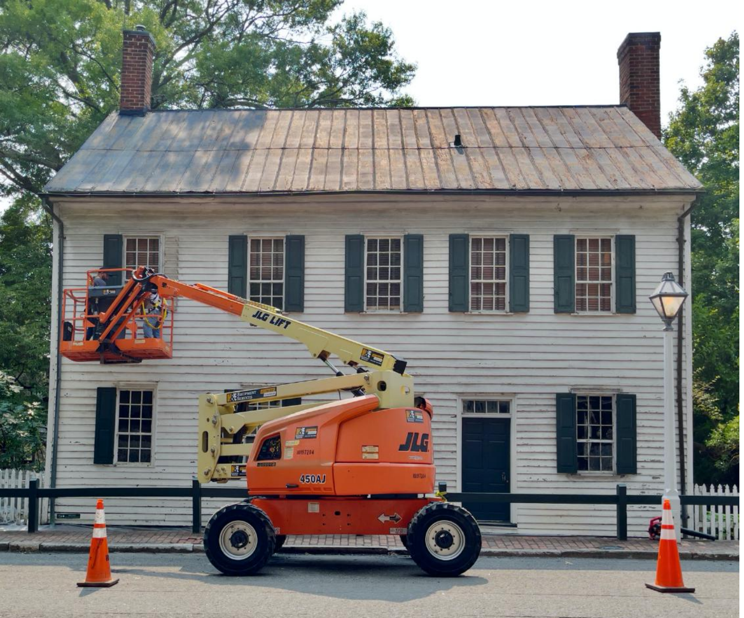
(Left to right) After removing the shutters, careful evaluation of the condition suggested repairs that were needed. The shutter repairs were primarily completed by joiner Ben Masterson with the logistical assistance of Erik Skarzynski, Director of Facilities, and Tony Bragg, Facilities Associate.
