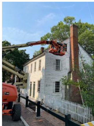
(Left to right) The Blum House, a basic white wood box, looks deceptively simple. The restoration work to the Blum House involved several layers of delicate restoration work; 1. Wood rot and repair to various elements (eaves, shutters, window sashes), 2. Exterior scrapping, priming, and painting, 3. And patching several roof leaks. The final result (photograph below) brings the house and attached print shop back to a crisp white painted finish with operable shutters.
