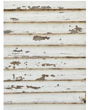
(Left to right) The Blum House, a basic white wood box, looks deceptively simple. The restoration work to the Blum House involved several layers of delicate restoration work; 1. Wood rot and repair to various elements (eaves, shutters, window sashes), 2. Exterior scrapping, priming, and painting, 3. And patching several roof leaks. The final result (photograph below) brings the house and attached print shop back to a crisp white painted finish with operable shutters.
