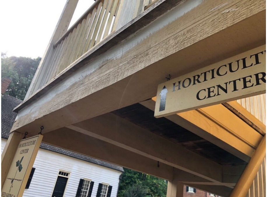
(TOP/BOTTOM - Left to right) The top row of photographs shows the extent of rot in the floor structure of the Main Street Porch. The floorboards were floating, unattached to the rotten beam below. The expert repairs and restoration work was completed by joiner Ben Masterson with the logistical assistance of Erik Skarzynski, Director of Facilities . The bottom row shows the removal of the floorboards which exposed the extent of the decay to the structure below. The finished repairs are blended in with the pre-existing building fabric and are awaiting repainting.
