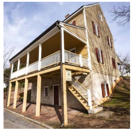
(Left to right) The Herbst House restoration and repair has a long list of needs. The most urgent needs are found on the Main Street façade. Visitors use the porch and sidewalk stairs to access the new SEED SAVING LAB, so these repairs are essential to ensure a good quality experience. The windowsills, bottom clapboard, and roof shakes all needed full replacement before re-painting could occur.
