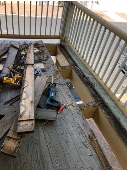
(TOP/BOTTOM - Left to right) The top row of photographs shows the extent of rot in the floor structure of the Main Street Porch. The floorboards were floating, unattached to the rotten beam below. The expert repairs and restoration work was completed by joiner Ben Masterson with the logistical assistance of Erik Skarzynski, Director of Facilities . The bottom row shows the removal of the floorboards which exposed the extent of the decay to the structure below. The finished repairs are blended in with the pre-existing building fabric and are awaiting repainting.
