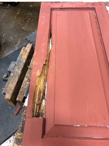
(left/right) Additional wood restoration work was needed on shutters and window sashes. The expert repairs and restoration work was completed by joiner Ben Masterson with the logistical assistance of Erik Skarzynski, Director of Facilities .
