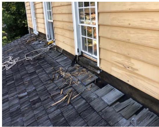
(Left to right) The Herbst House restoration and repair has a long list of needs. The most urgent needs are found on the Main Street façade. Visitors use the porch and sidewalk stairs to access the new SEED SAVING LAB, so these repairs are essential to ensure a good quality experience. The windowsills, bottom clapboard, and roof shakes all needed full replacement before re-painting could occur.
