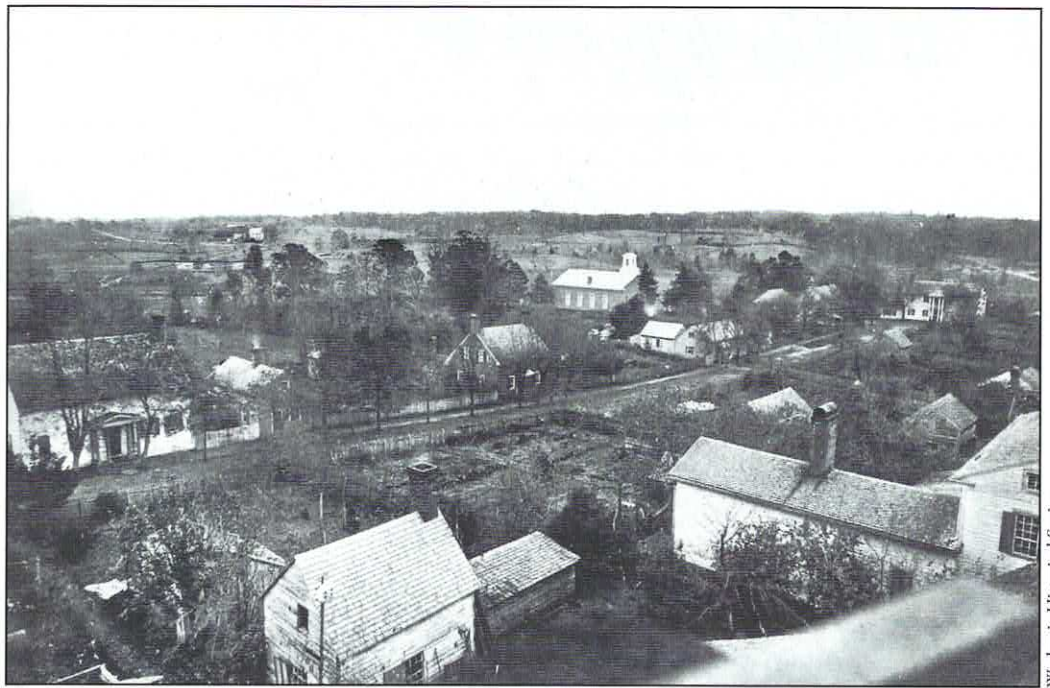
View southeast across Salem, ca. 1865, to background landscape that will become Happy Hill in 1872.
