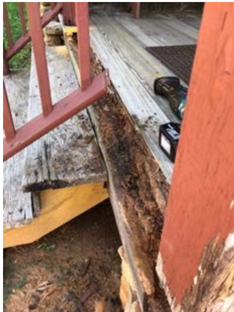
(Left to right) The next Fresh Coat Initiative project is the Log Church (the first church building built for enslaved Afro-Moravians). Initial analysis has revealed a high level of rot and deterioration to not only the structural porch beams but also the dry stack foundation piers. Seeing this level of need has placed the Log Church at the top of our priority list. The expert repairs and restoration work is being completed by craftsman Ben Masterson, residents Bill Tobiassen and Doug Williams with the logistical assistance of Erik Skarzynski, Director of Facilities and his team.
