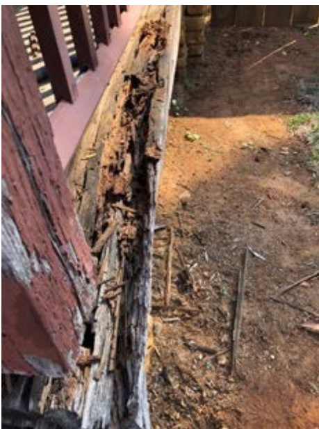
(Left to right) The next Fresh Coat Initiative project is the Log Church (the first church building built for enslaved Afro-Moravians). Initial analysis has revealed a high level of rot and deterioration to not only the structural porch beams but also the dry stack foundation piers. Seeing this level of need has placed the Log Church at the top of our priority list. The expert repairs and restoration work is being completed by craftsman Ben Masterson, residents Bill Tobiassen and Doug Williams with the logistical assistance of Erik Skarzynski, Director of Facilities and his team.
