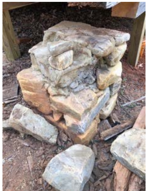
(Left to right) The next Fresh Coat Initiative project is the Log Church (the first church building built for enslaved Afro-Moravians). Initial analysis has revealed a high level of rot and deterioration to not only the structural porch beams but also the dry stack foundation piers. Seeing this level of need has placed the Log Church at the top of our priority list. The expert repairs and restoration work is being completed by craftsman Ben Masterson, residents Bill Tobiassen and Doug Williams with the logistical assistance of Erik Skarzynski, Director of Facilities and his team.
