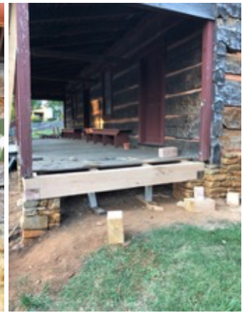
(Left to right) The Log Church for the Enslaved (Reproduction c. 1999), Wood rot on the porch structure, restoration in process showing new structure in place. The expert repairs and restoration work is being completed by craftsman Ben Masterson, residents Bill Tobiasen and Doug Williams with the logistical assistance of Erik Skarzynski, Director of Facilities, and his team.
