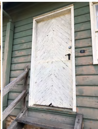
(Left to right) Anna Catharina House c. 1771-72 (Reconstruction c. 1954). Every surface of the structure needed scraping, priming, and paint. The expert repairs and restoration work was completed by craftsman Ben Masterson, with the logistical assistance of Erik Skarzynski, Director of Facilities, and his team.
