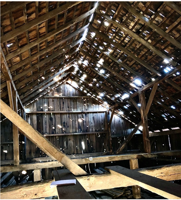
The Voltz Barn needed attention. Sunlight poked through the decaying wood shake roof, and the holes in the roof allowed water to infiltrate and rot important structural members.
