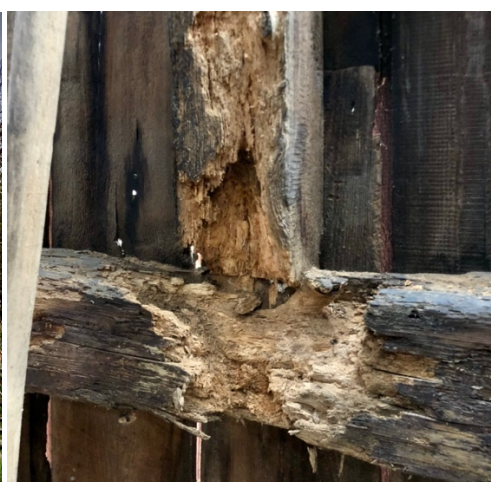
A photograph showing the original location of the barn structure, the Voltz Barn roof being installed, rot damage to the structure.
