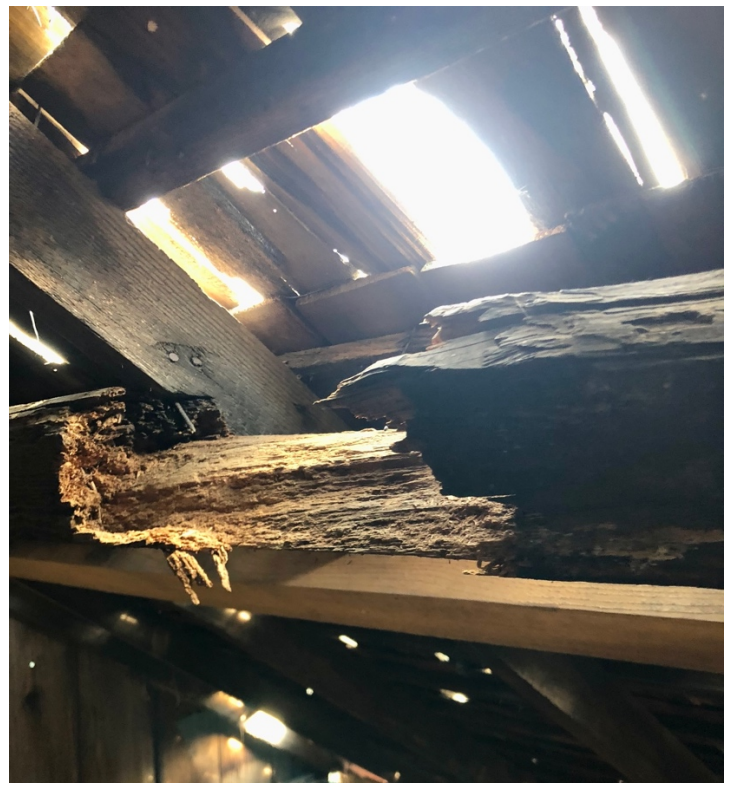
The Voltz Barn needed attention. Sunlight poked through the decaying wood shake roof, and the holes in the roof allowed water to infiltrate and rot important structural members.
