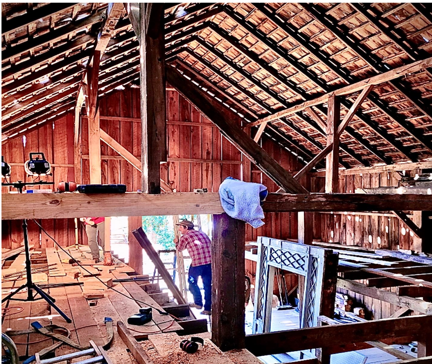
Ben Masterson, Restoration Carpenter, is shown working in the Voltz Barn restoring the highly detailed timber connections.
