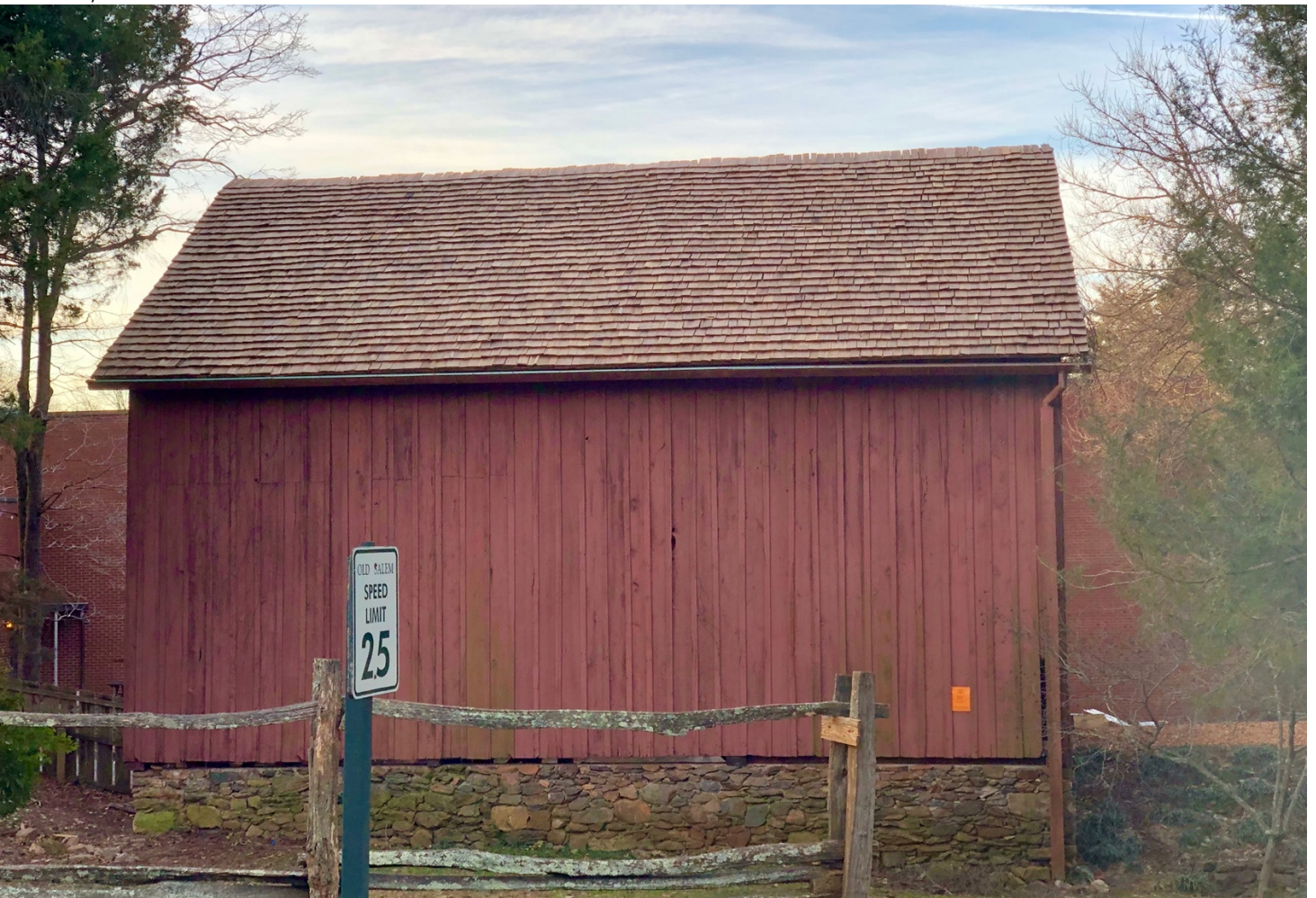
The Voltz Barn showing the newly completed wood shake roof. This roof was approved by the Historic Resources Commission and will provide decades of protection for the newly restored timber structure.
